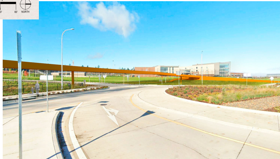
Alignment A2 - West Landing
